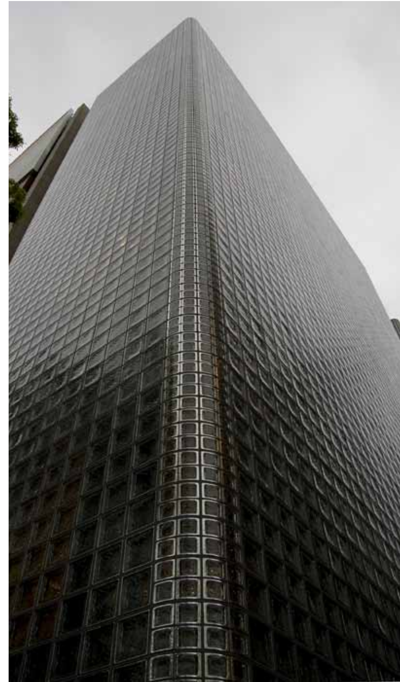
Renzo Piano's Hermes Building in Tokyo has a façade of glass block. Photo: Mariano Colantoni
