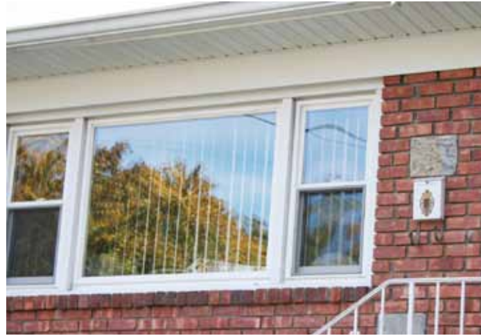
Reflections on home windows are a significant source of bird mortality. The partially opened vertical blinds seen here may break up the reflection enough to reduce the hazard to birds. Photo: Christine Sheppard, ABC
