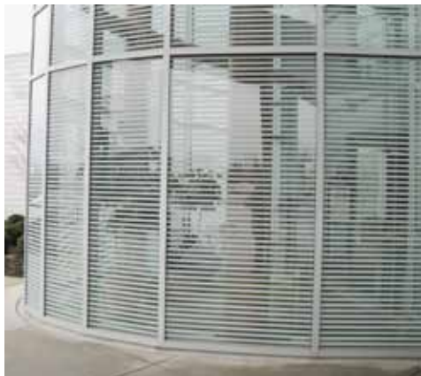
Dense stripes of internal frit on University Hospital's Twinsburg Health Center in Cleveland, by Westlake, Reed, Leskosky will overcome virtually all reflections. Photo: Christine Sheppard, ABC
