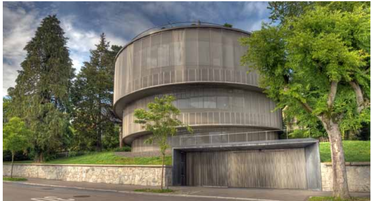
The steel mesh enveloping Zurich's Cocoon in Switzerland, designed by Camenzind Evolution Ltd, provides privacy and protects birds, but still permits occupants to see out. Photo: Anton Volgger
