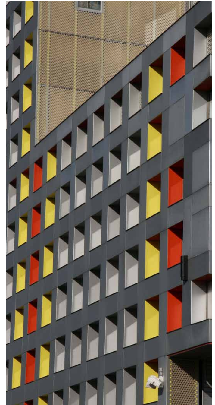
Deeply recessed windows, such as these on Stephen Holl's Simmons Hall at MIT, can block viewing of glass from most angles. Photo: Dan Hill
