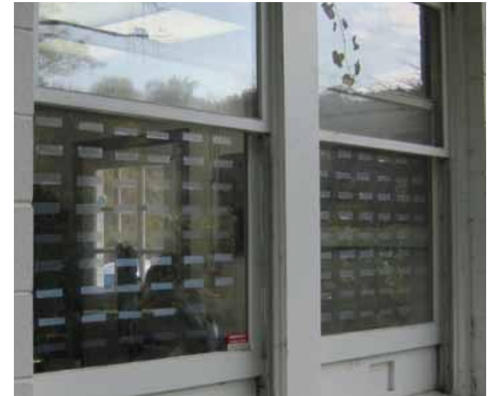
Tape decals (Window Alert shown here) placed following the 2 x 4 rule can be effective at deterring collisions. Photo: Christine Sheppard, ABC
