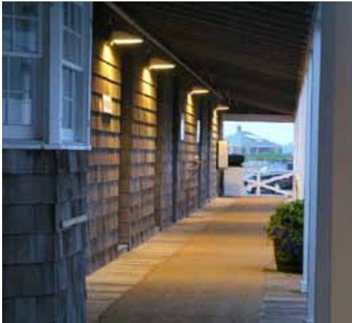
Shielded lights, such as those shown above, cut down on light pollution and are much safer for birds. Photo: Susan Harder
