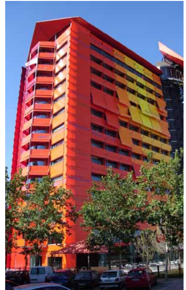
The Hotel Puerta America in Mexico City was designed by Jean Nouvel, and features external shades. This is a flexible strategy for sun control, as well as preventing collisions; shades can be lowered selectively when and where needed. Photo: Ramon Duran
