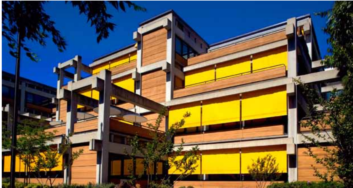
External shades, as shown here on the Batson Building in Sacramento, California, designed by Sym Van der Ryn, are a simple and flexible strategy for reducing bird collisions, as well as controlling heat and light. Photo courtesy of MechoShade
