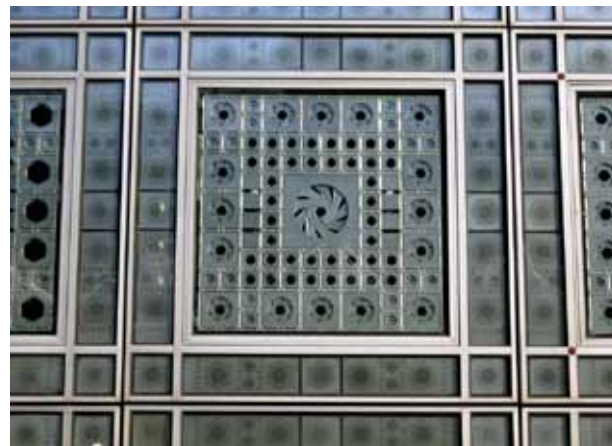
Instead of glass, this side of Jean Nouvel's Institute Arabe du Monde in Paris, France features motor-controlled apertures that produce filtered light in the interior of the building. Photo: Vicki Paull
