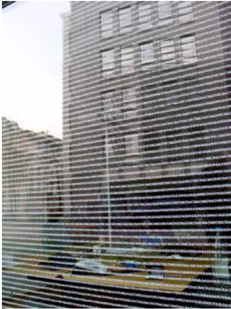
The glass facade of SUVA Haus in Basel, Switzerland, renovated by Herzog and de Meuron, is screen-printed on the outside with the name of the company owning the building. Photo: Miguel Marqués Ferrer
