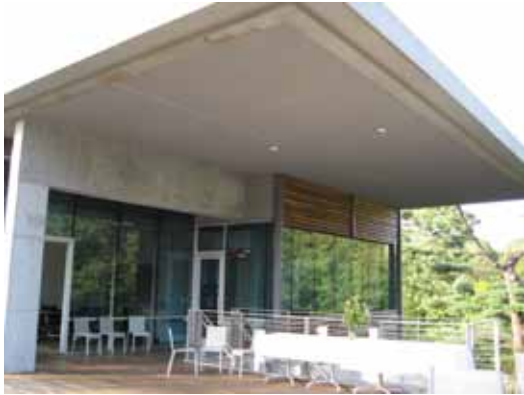
Overhangs block viewing of glass from some angles, but do not necessarily eliminate reflections. Photo: Christine Sheppard, ABC
